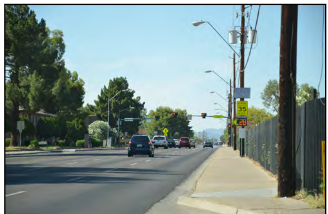
Bike lanes do not exist between SR-101 and Thunderbird Road (looking north approaching Thunderbird High School)
