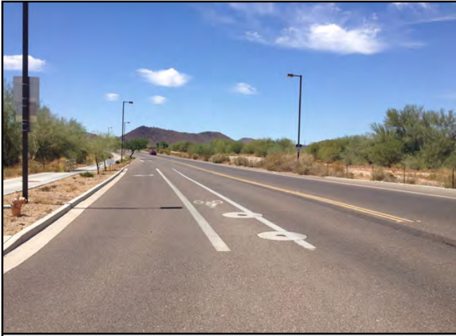
Looking West out of Reach 11
