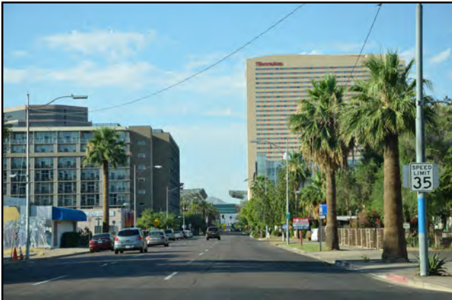
3rd Street south of Roosevelt One Way section (looking south)
