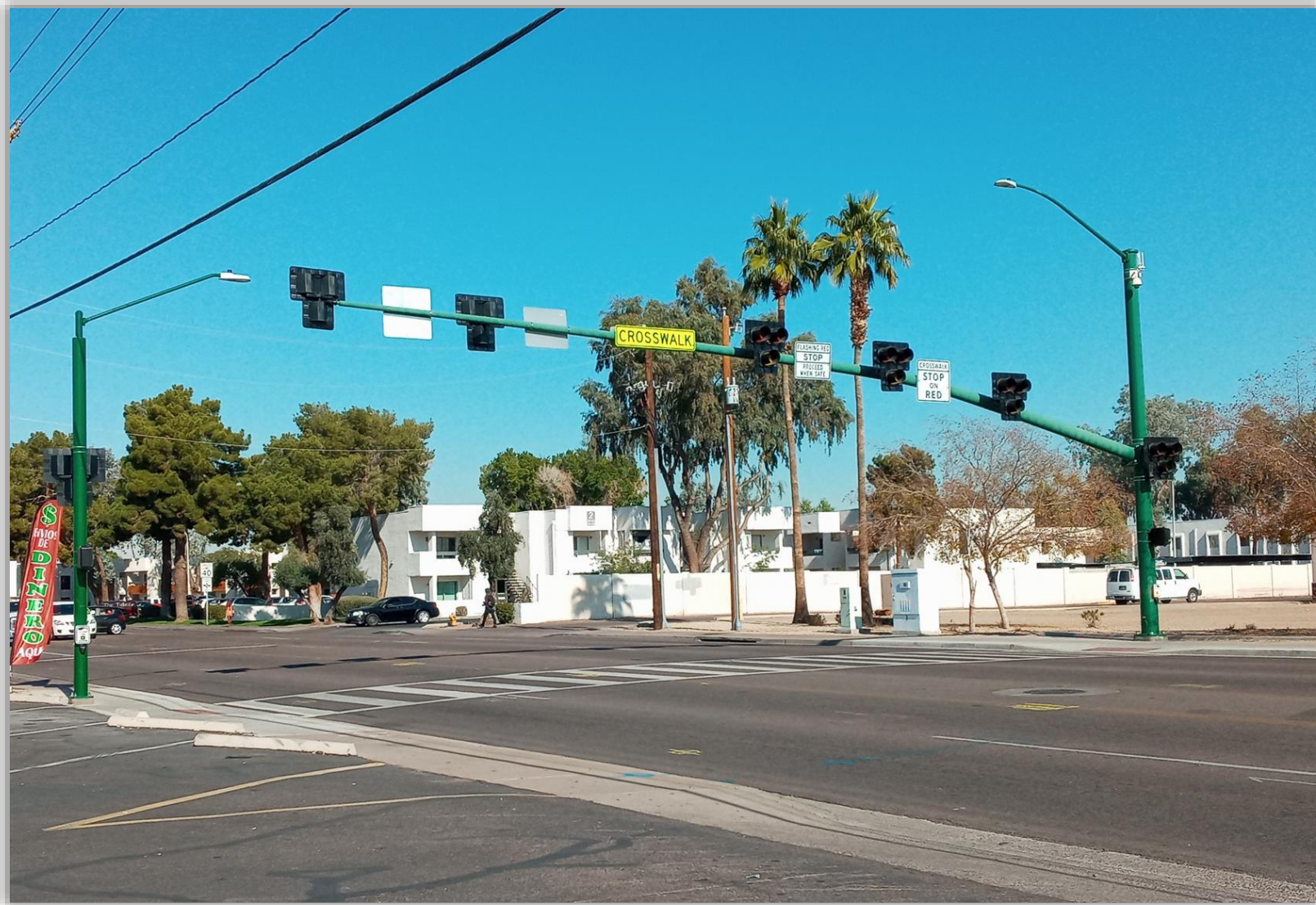
The Hawk Signal at 6104 N 27th Avenue was Activated in December of 2021.
