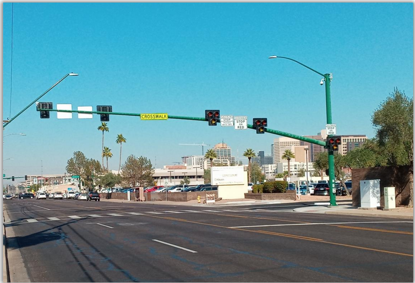
The Hawk Signal at 1215 South 7th Avenue was Activated in October of 2021.
