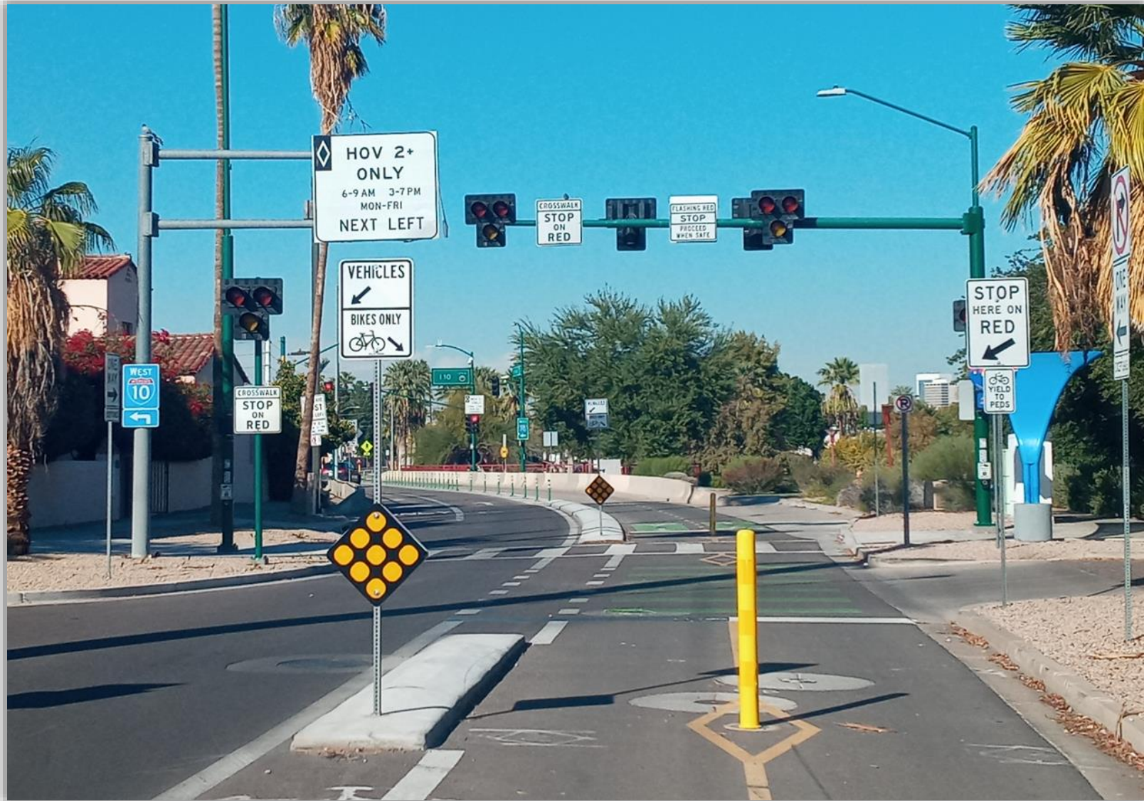
The Hawk Signal at 3 rd Avenue and Latham Street was Activated in June of 2021.
