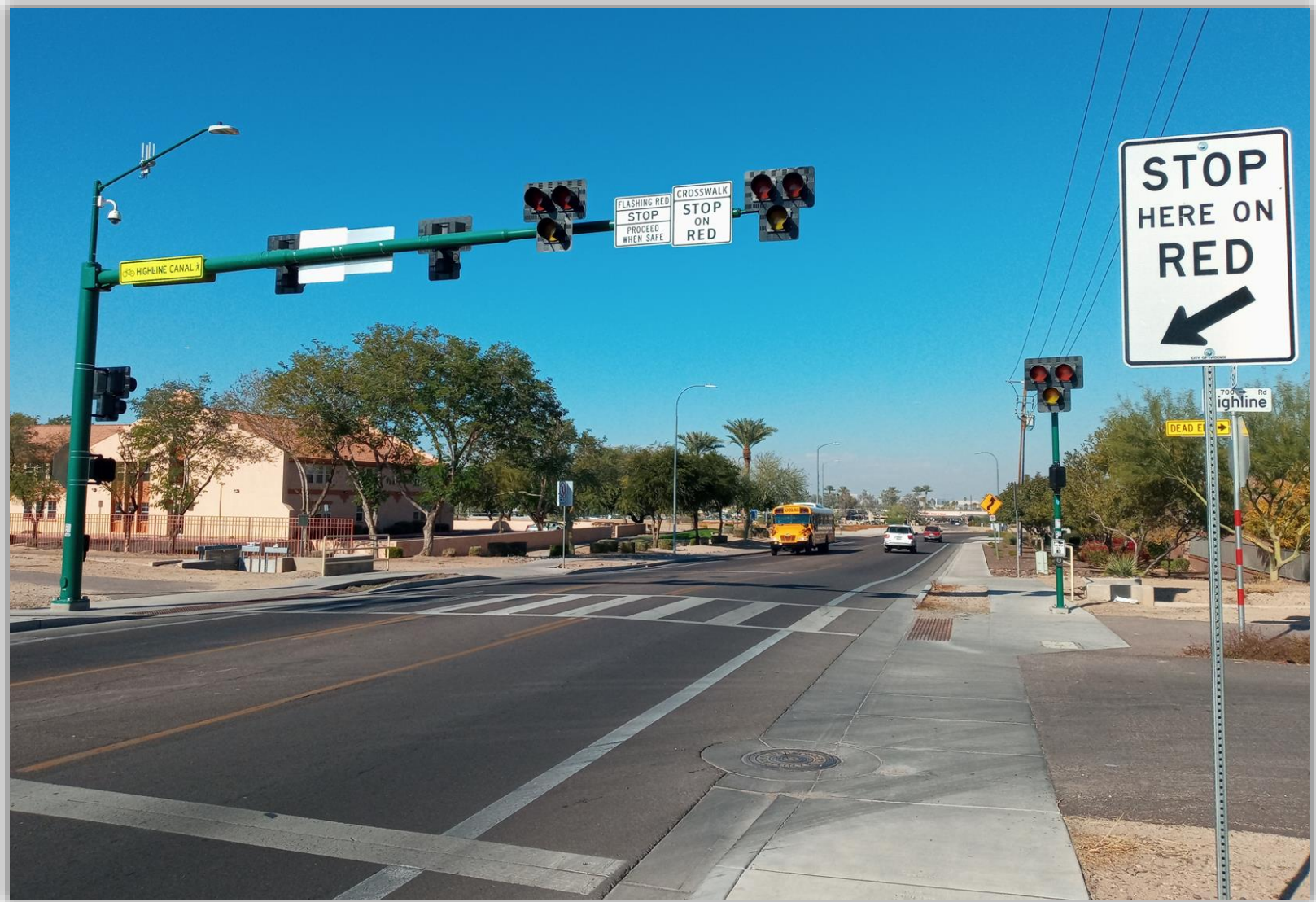
The Hawk Signal at 8025 South 7th Street (Highline Canal) was Activated in January of 2021.
