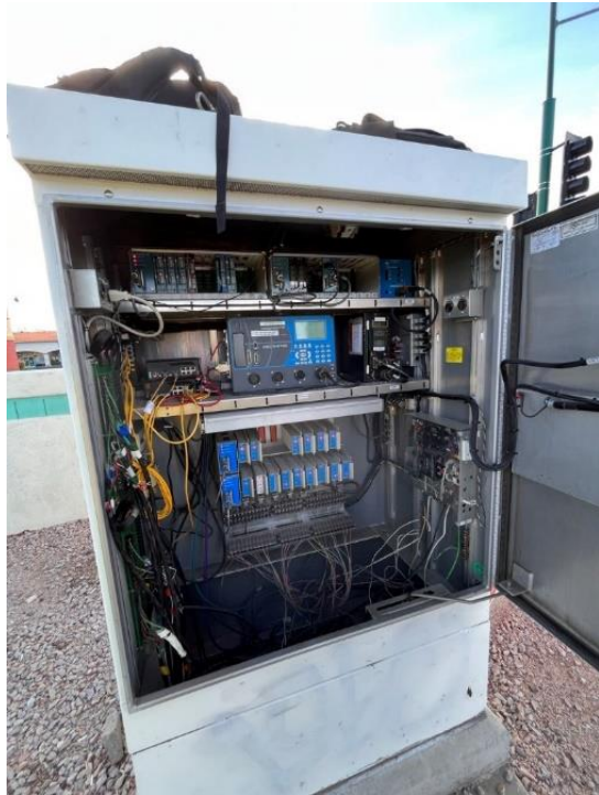
Figure 3.3 a) Miovision's smartview camera installed sensors, b) Traffic control cabinet & conduit
