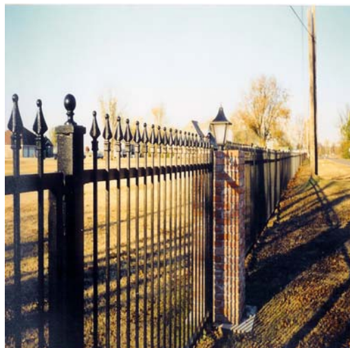
Wrought-iron fencing (Figure 3)
