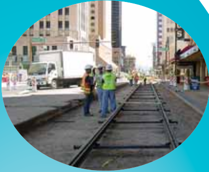
Light rail track construction in Downtown
