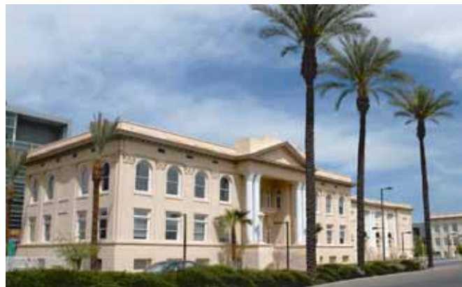
Renovation of the Phoenix Union High School historic buildings for the University of Arizona Medical School.
