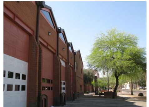
Fire station on 4th Avenue north of Van Buren
