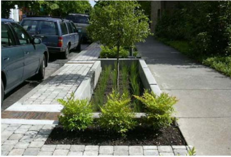
Landscaped drainage troughs (12 th & Montgomery, Portland, Oregon)
