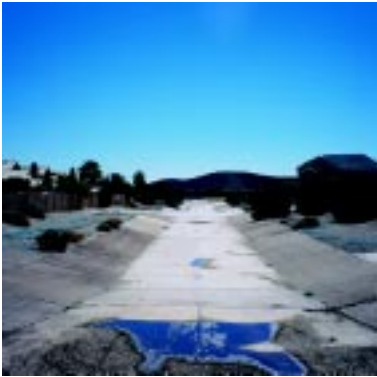
Figure 3.29 Wash corridor lined with concrete provides minimal benefit as open space to either wildlife or the public
