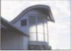
The turbine housing roof is a cap that can be lifted to remove and service the turbine inside. The artist has designed a shadow device installed in the generator room to project the shadows of three wave patterns on the curved window, whenever the generator is online producing electricity.
