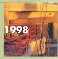
Thunderbird Road Vehicular Bridge Beth Galston
