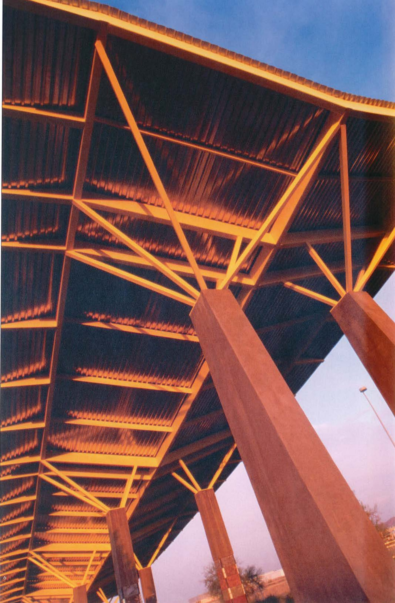
Designed by Orcutt/Winslow, landscape architect Christy Ten Eyck and artist Tom Strick, the Rio Salado Gateway is the first completed element of the Rio Salado Habitat Restoration project first envisioned more than 30 years ago at Arizona State University. (opposite page) Several rare views of the Salt River with native water flow following heavy rainfall. The viceroy is normally dry as a result of the construction of Roosevelt Dam in 1903.
