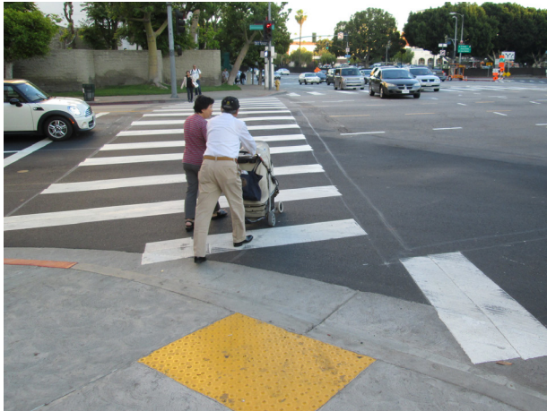
Not recommended: Diagonal curb ramp configuration.
