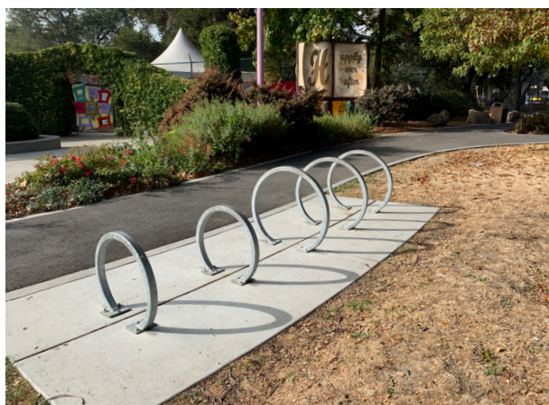
Racks with square tubing, good spacing, and a concrete base likewise offer two points of contact.
