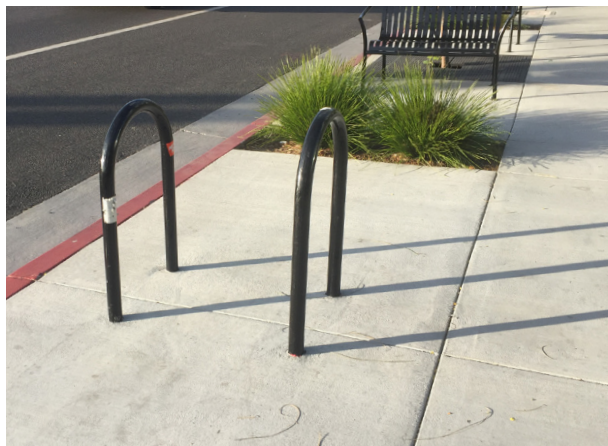
Inverted-U racks provide two points of contact.
