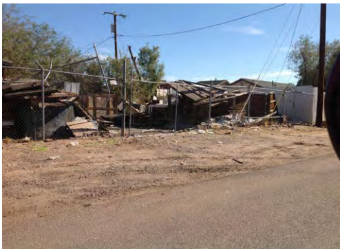
Deterioration of Site
