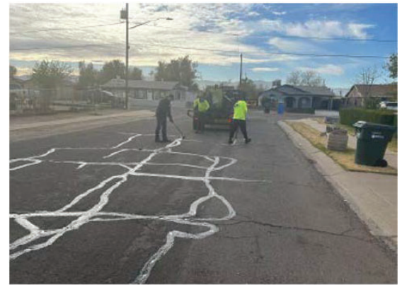
Crack Seal
