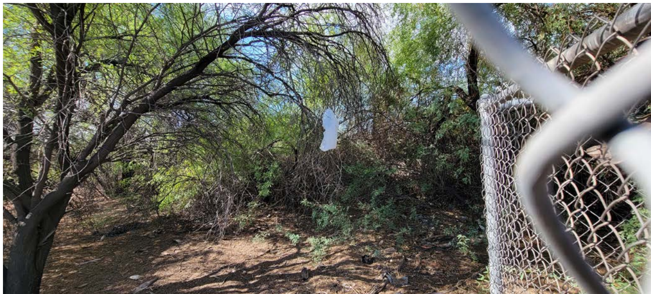
FIGURE BB: OVERGROWN VEGETATION
