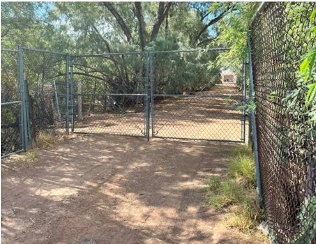
FIGURE E: THOMAS ROAD ACCESS GATE
