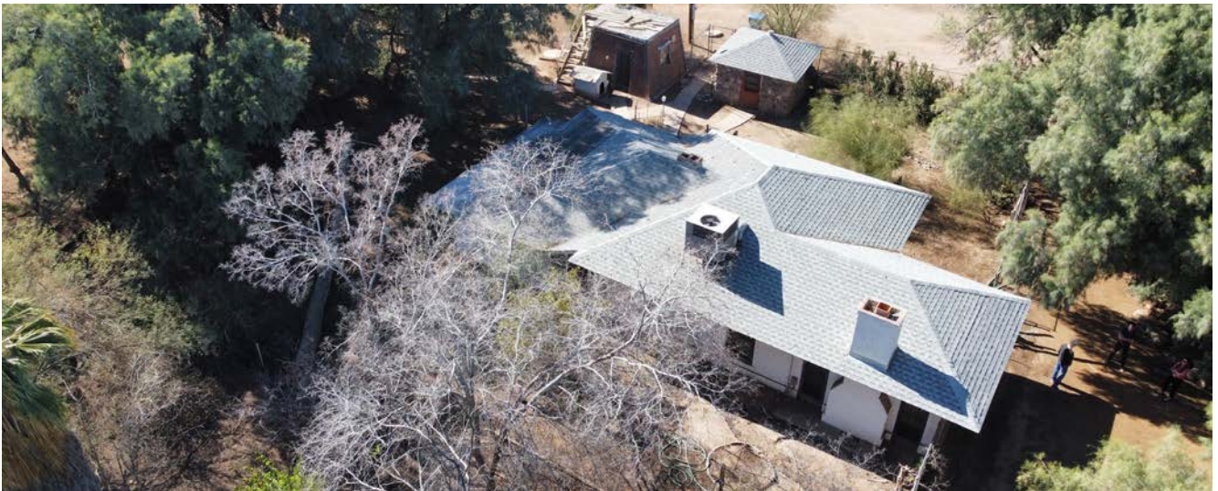
FIGURE DD: DETERIORATING STRUCTURES
