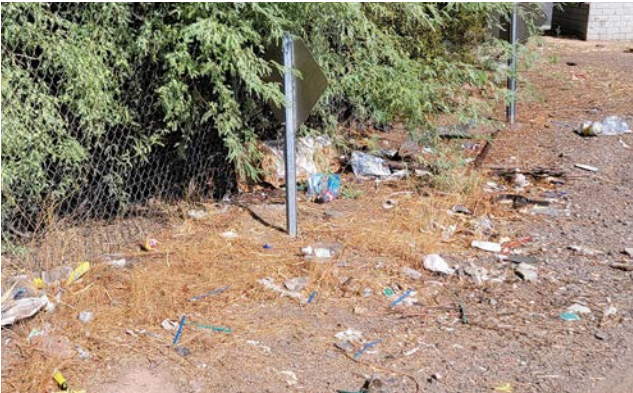
FIGURE J: TRASH AND DEBRIS
