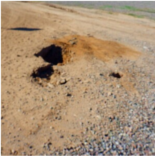
Hole/washout on site
