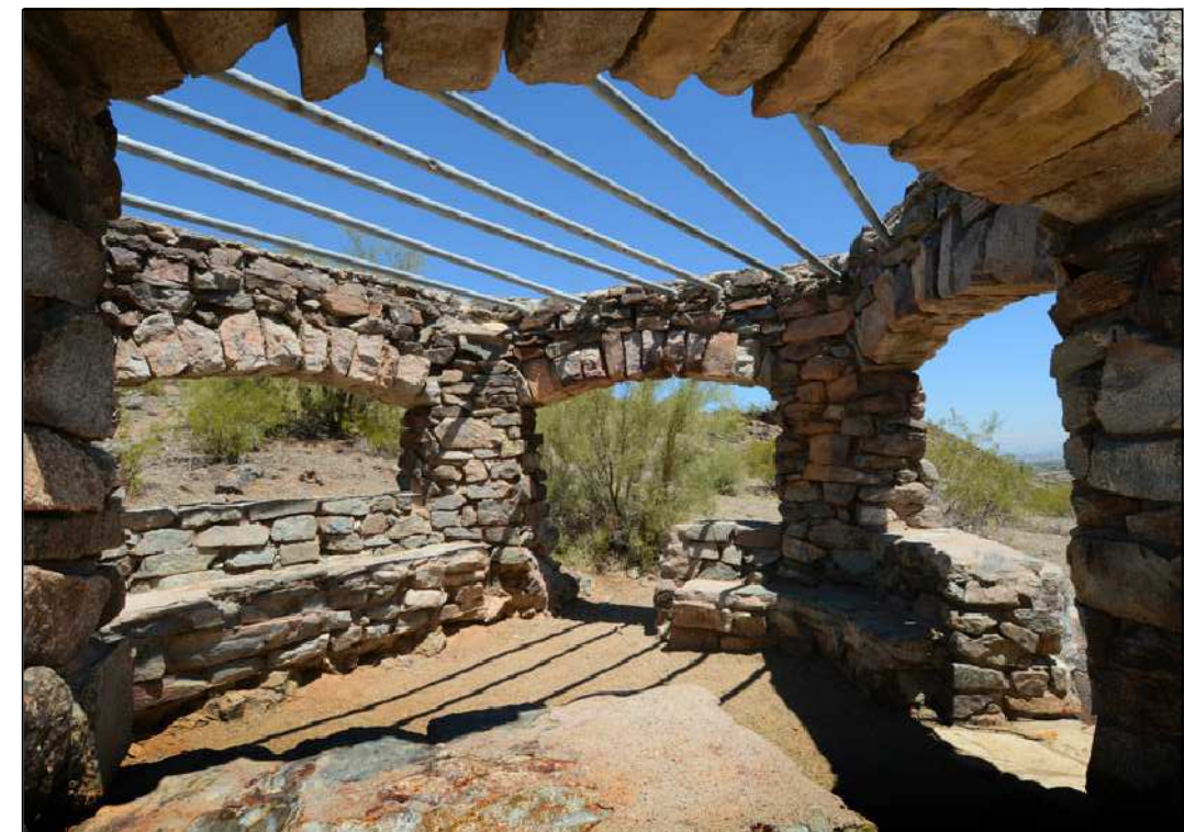
Photograph looking at steel pipe lattice
