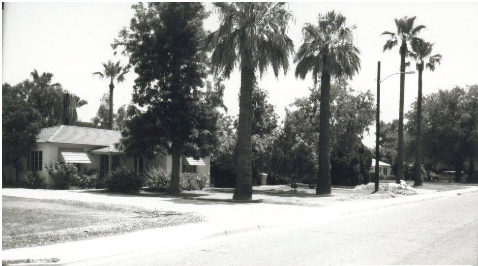
14-32-2 Villa Potero 2801 N 21st St to SE Phx Pre-1950 Recon (6:23)
