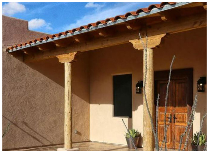
Exposed timber used for columns, beams, and rafters. Curved roof tiles. Warm natural earth tones. Shaded or inset windows.
