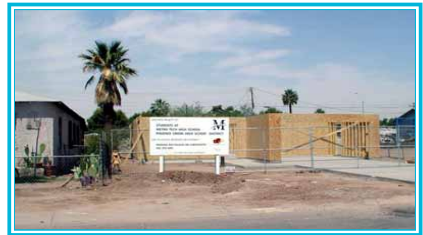
Figure 23 - Housing under construction
