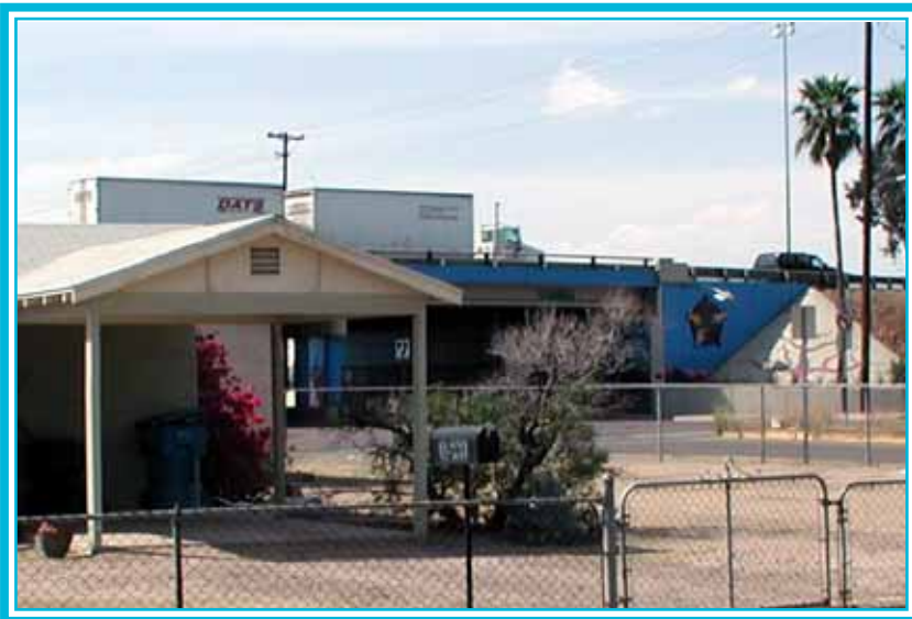
Figure 29 - Elevated freeway (in background)
