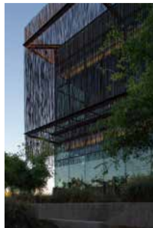
Street and river-oriented buildings
