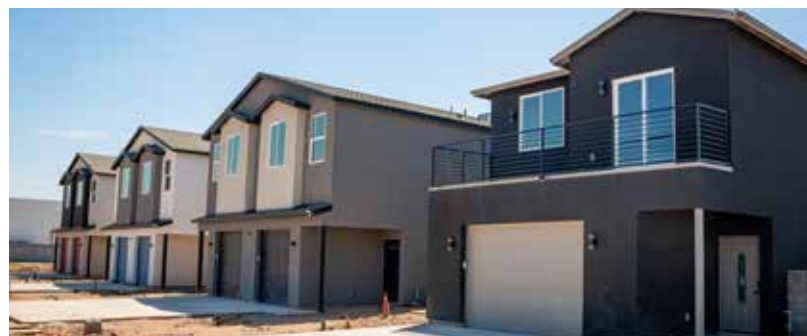
New homes under construction near 28th Street and Wood Street Source: Bloomberg Philanthropies
