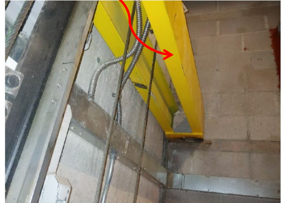
Picture 2: The same "dead" side that holds the side of the cables that do not move. This beam installed by the elevator manufacturer is supported by the hoistway wall. It is doubted this load was communicated to the building designer. This hoistway consists of both masonry and concrete walls.
