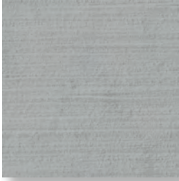
Light Broom Finished TILT-UP CONCRETE EXAMPLE
