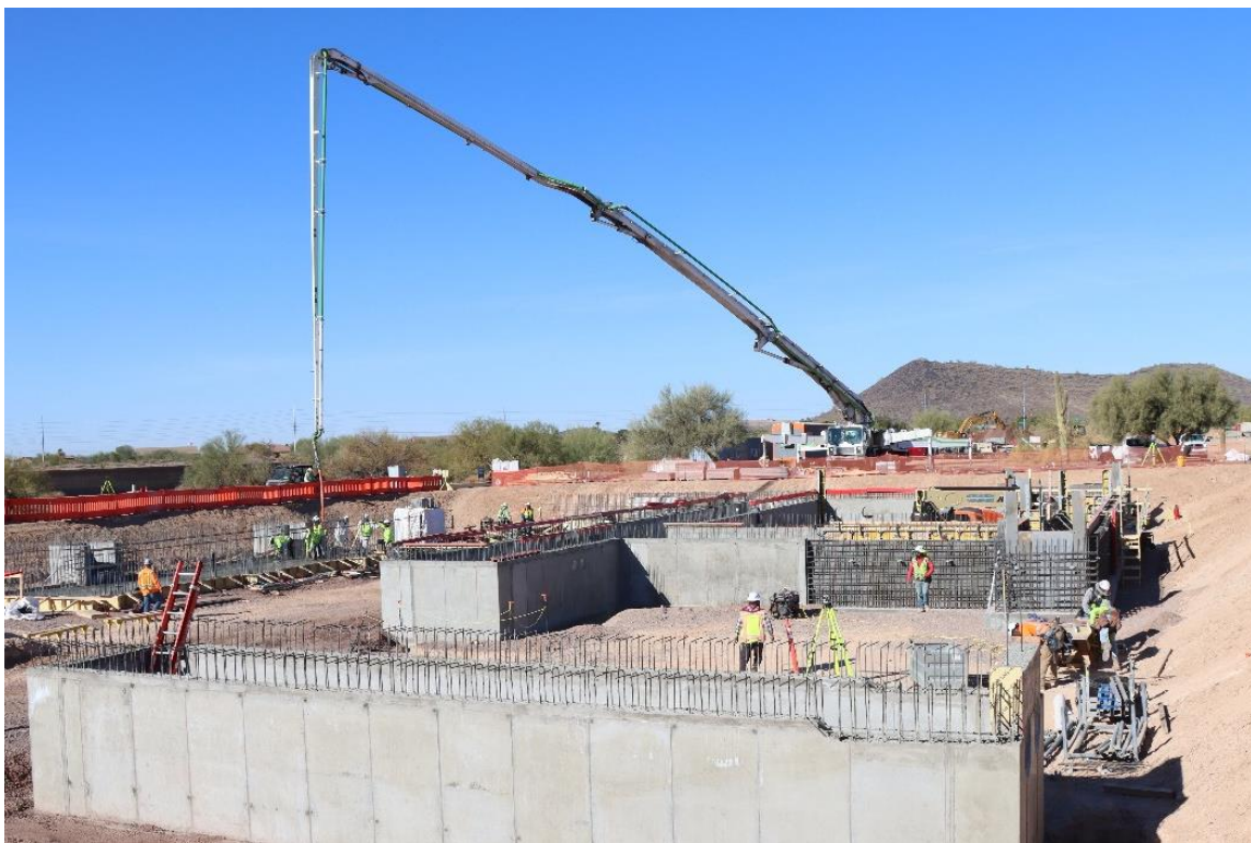
New facilities being built at the Cave Creek plant.
