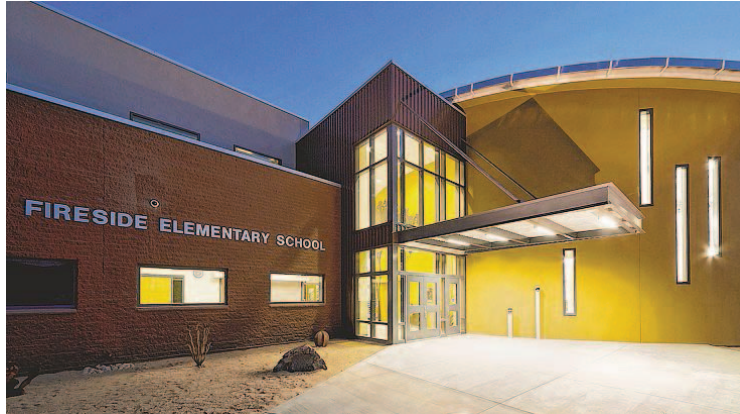
Fireside Elementary School in the Paradise Valley Unified School District is designed to use 55 percent less energy than comparable buildings in the area. It also strives to produce and conserve as much energy and water as it consumes. PHOTOS BY ARIZONA FORWARD
