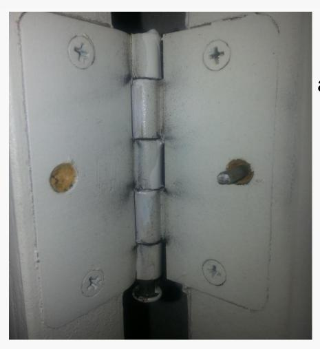
Drive screw or nail into door leaving it exposed about 3/8" to fit into hole drilled in door jam
