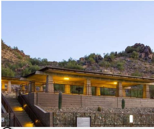
8 Refurbish Existing Ramada
