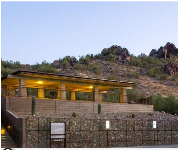
1 Refurbish Existing Ramada
