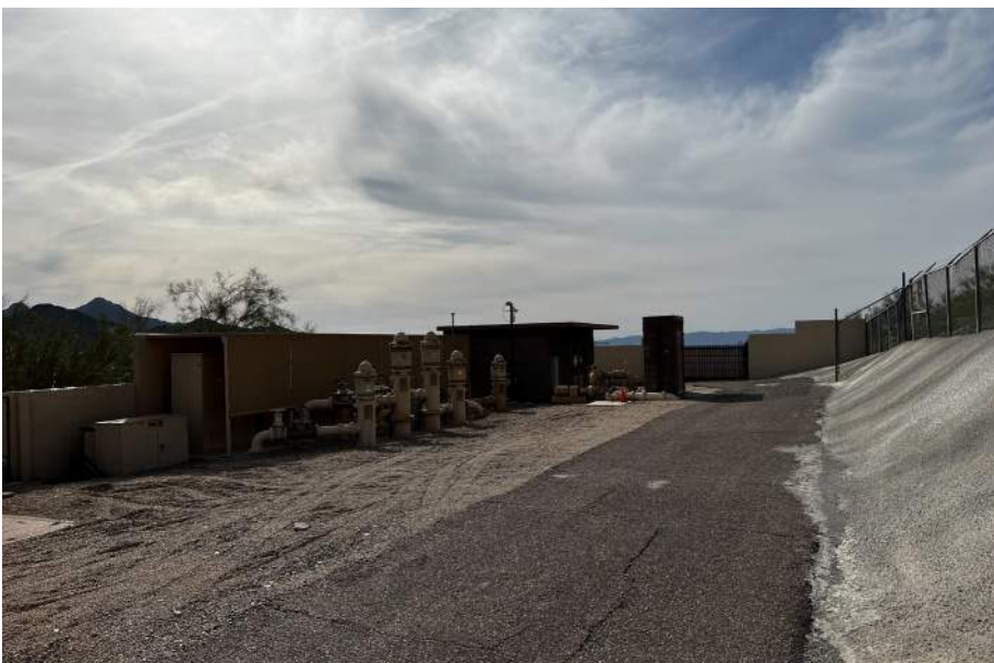
City of Phoenix Well Site
