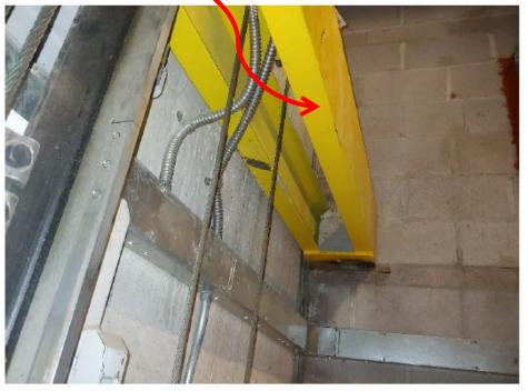
Picture 2: The same "dead" side that holds the side of the cables that do not move. This beam installed by the elevator manufacturer is supported by the hoistway wall. It is doubted this load was communicated to the building designer. This hoistway consists of both masonry and concrete walls.
