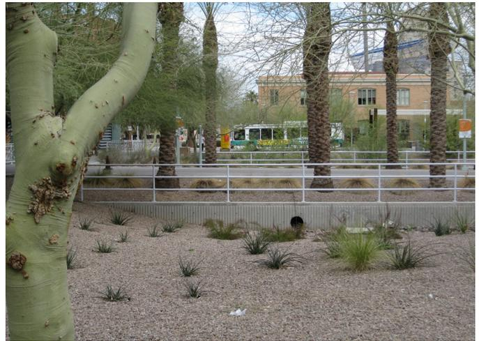
This investment contributes to permeability, and can be used to promote cooling. In general, properly designed and constructed retention cells achieve excellent removal of heavy metals, moderate storm water discharge, enhance wildlife habitats, and act as windbreaks and noise absorption.
