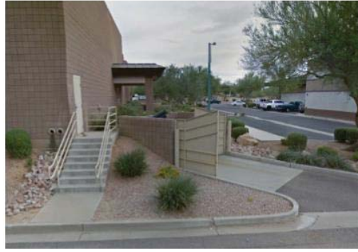
10. SOUTHEAST CORNER LOOKING EAST
