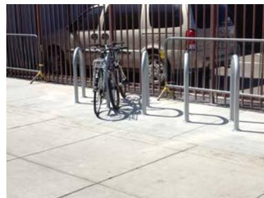
*Inverted-U racks are efficient and allow bicycles to be locked in an upright position utilizing standard U locks.*
