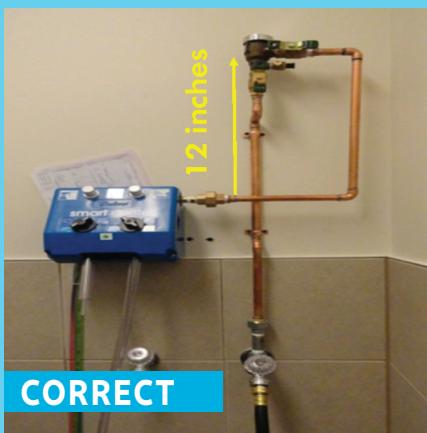
The waterline supply to the chemical dispenser must be either a designated line or can be connected behind the faucet (prior to the atmospheric vacuum breaker) that is currently being used.
