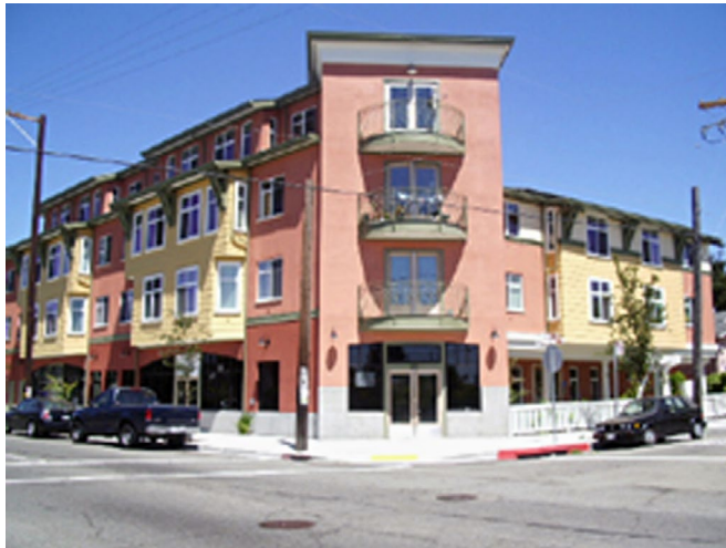
This affordable housing complex in Berkeley, California serves seniors with household incomes less than 30%, 50%, or 60% of the area median income. Source: bbiconstruction.com
