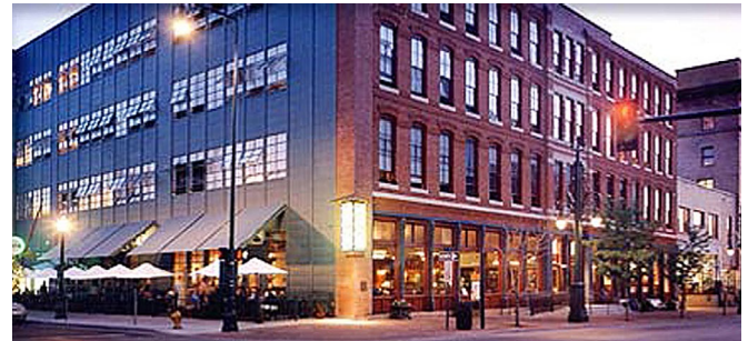
Mercantile Square in Denver, Colorado is a mixed-use space with a bookstore, restaurant, office space, and affordable rental housing funded through LIHTC.
