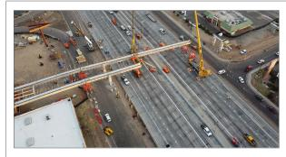
"Bridging East to West" Cranes set the final girders for the Northwest Extension, Phase II over I-17.
