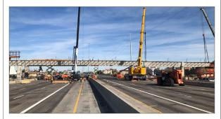
In March of this year construction crews completed bridge girder installation crossing over Interstate 17 for the Northwest Extension, Phase II.
