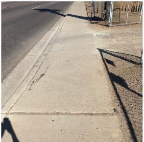
Photo 65 – Sidewalk not constructed in accordance with ADA Guidelines
