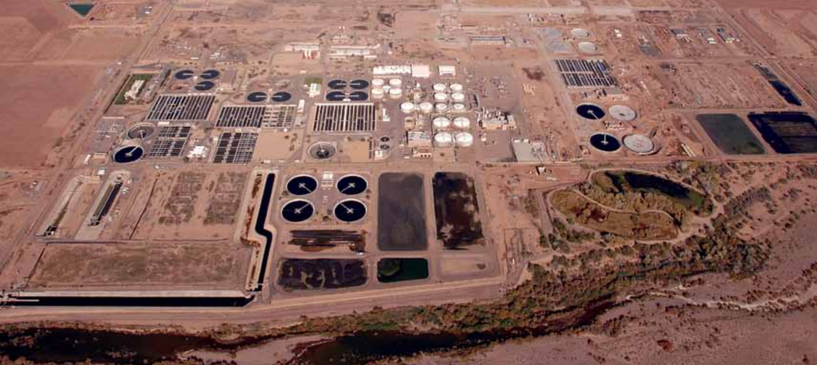
Figure 3. City of Phoenix 91 st Avenue Wastewater Treatment Plant.
