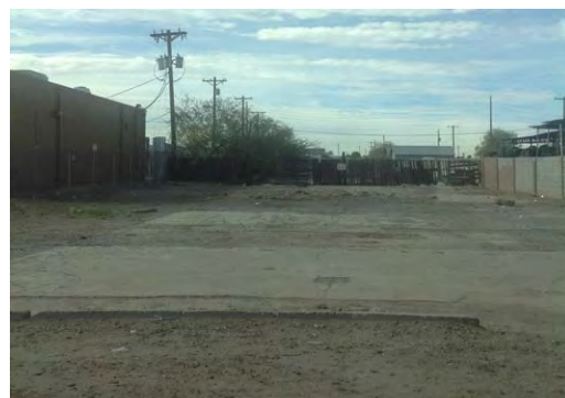
Partial Concrete Foundation
