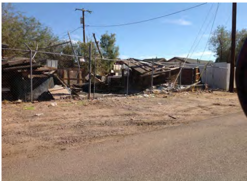
Deterioration of Site
