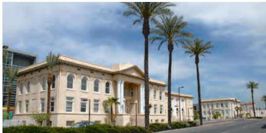
Renovation of the Phoenix Union High School historic buildings for the University of Arizona Medical School.
