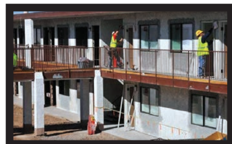
Collins Court Apartments, Under Construction
