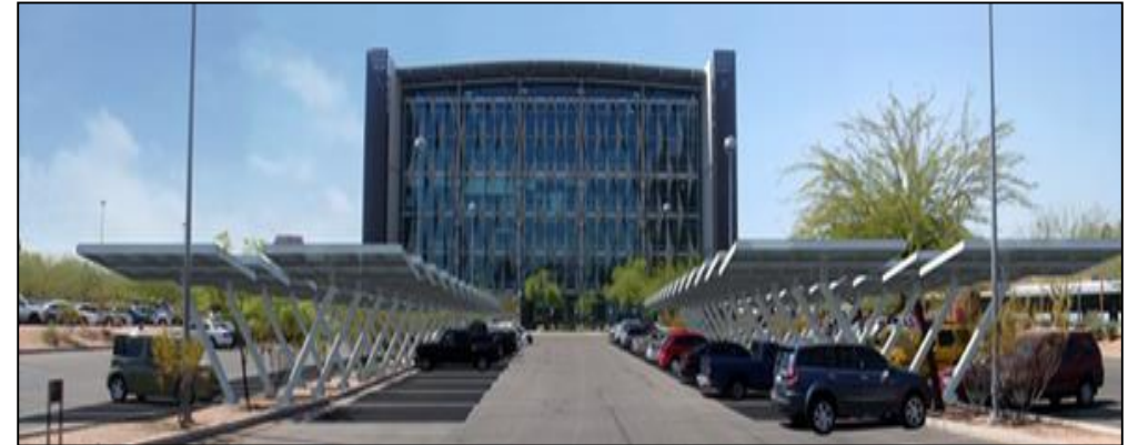
Burton Barr Library: 148 KW
