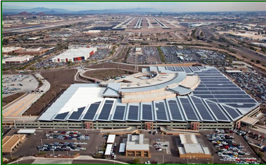
Rental Car Center Solar 4.2 Mega-watts
