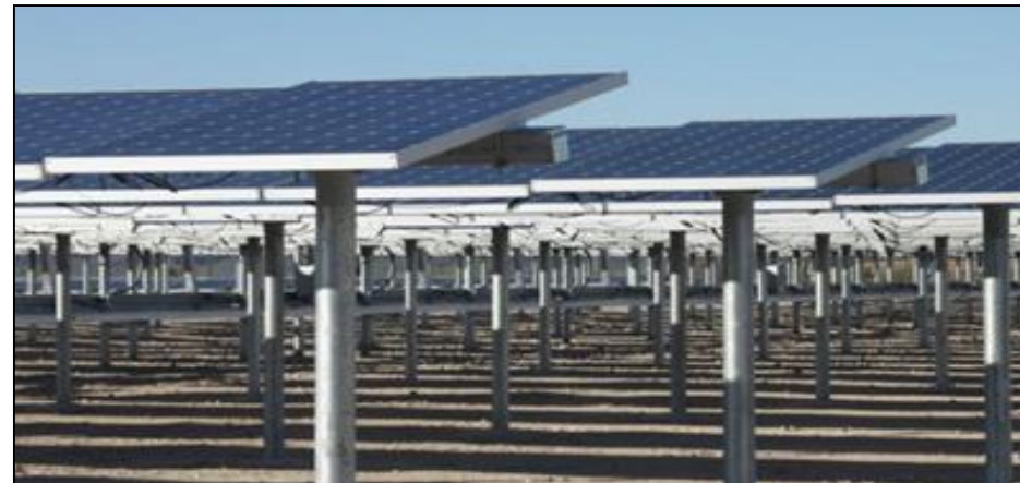
Lake Pleasant Water Treatment Plant – 7.5 MW
