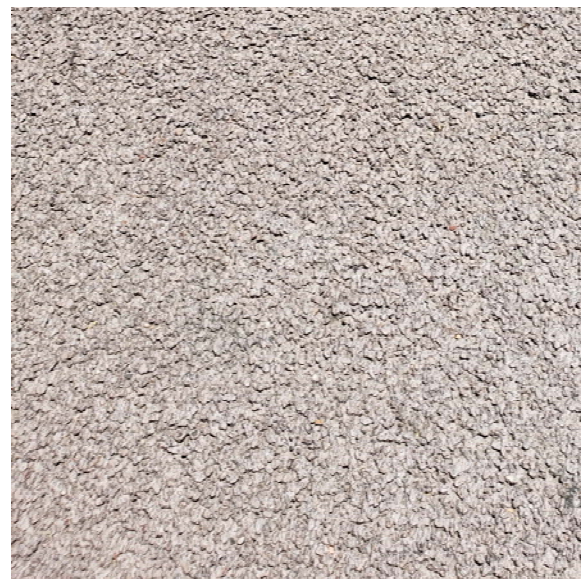
Pervious concrete at Central Station
