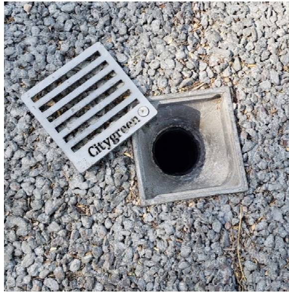
Unclogged drain inlet
