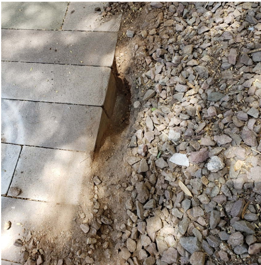
Grouted pavers around edge (header)
