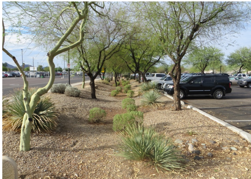
Union Hills Service Bioswale
