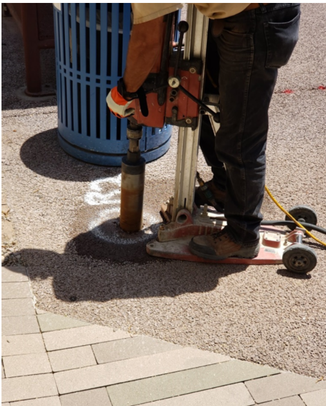
Pavement boring at Central Station
