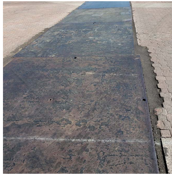
Trenching at intersection
