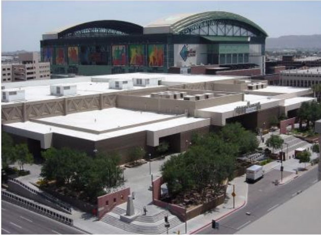
A white cool roof on the Phoenix Convention Center.
