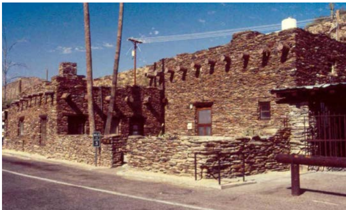
The Administration Building at the entrance to South Mountain Park was constructed in 1934 by the Civilian Conservation Corps, one of the most ambitious and far-reaching New Deal programs implemented during the Great Depression. The Pueblo Revival-style building is a romantic interpretation of a Hopi pueblo designed to comfortably blend within the natural park environment utilizing local schist stone and roof heights that lift and drop like the surrounding mountains.
