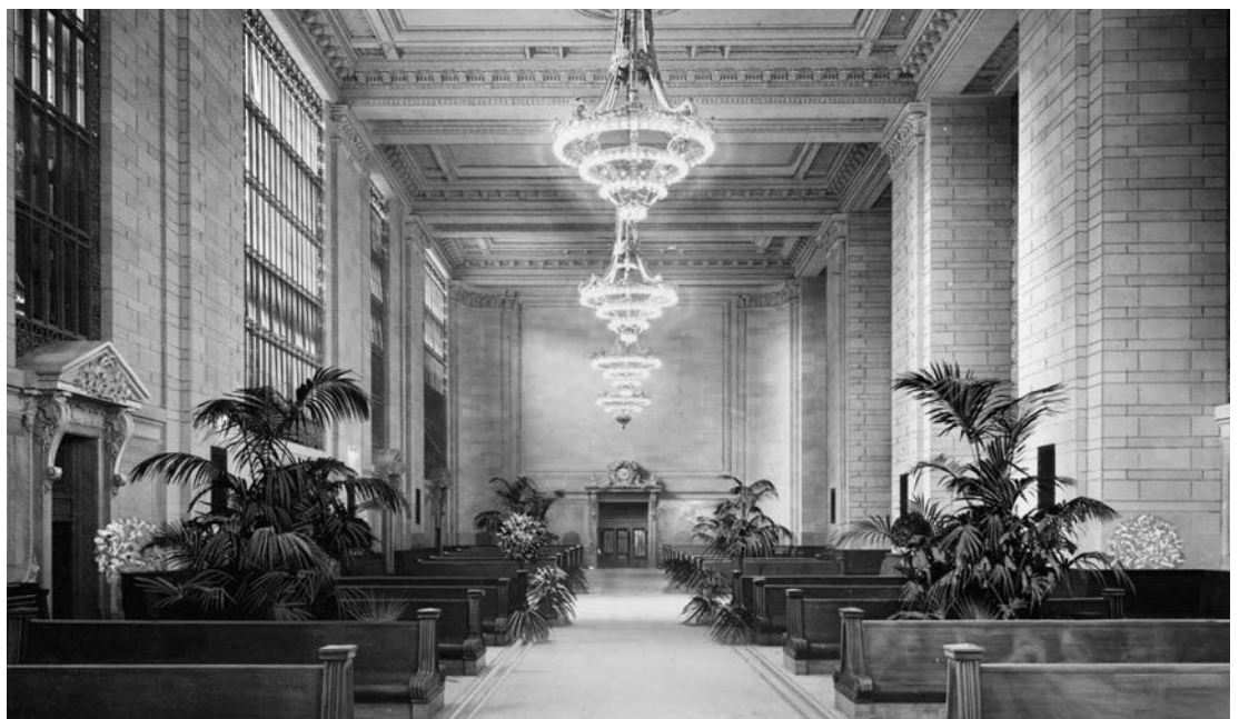
Photo of the main waiting room of Grand Central Terminal in New York City taken between 1910 and 1920; Photo courtesy of Library of Congress, LC-DIG-det-4a24549.
