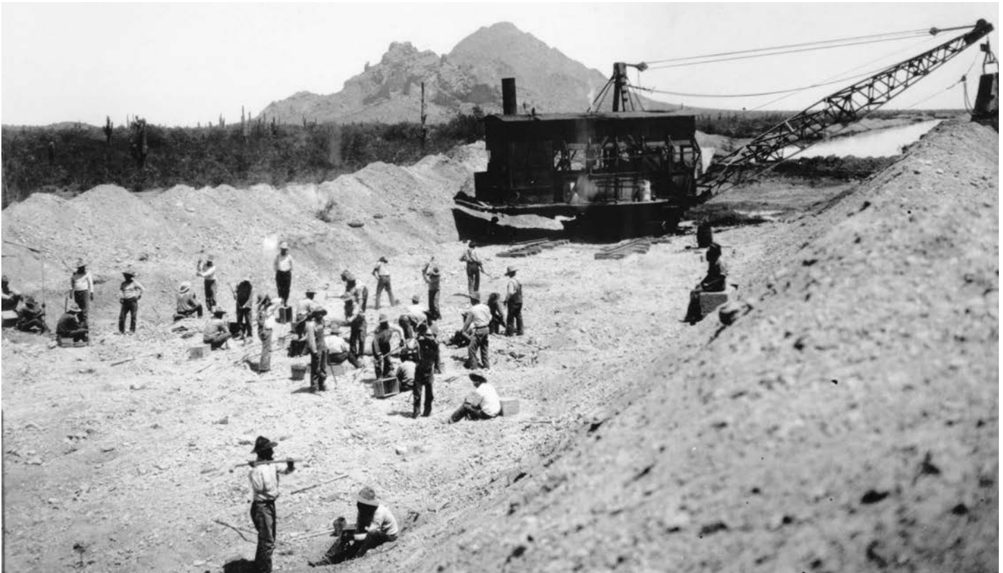
The Arizona Canal was begun in 1883. In the fall of 1907 the Arizona Canal was enlarged with a Bucyrus dredger placed on a boat. Over 113,000 cubic yards of material was removed and reused to build a road on the south side of the canal. Photo courtesy Library of Congress, Prints & Photographs Division, HAER, Reproduction number HAER ARIZ,7-PHEN.V,1--4
