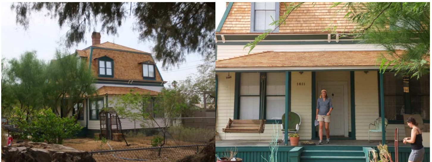
These photos from 2013 show the rehabilitation of the Tweed House's wood shingle roof and many of the windows.
