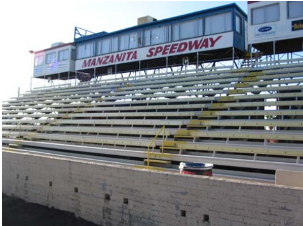
View of center stands, looking northwest.
