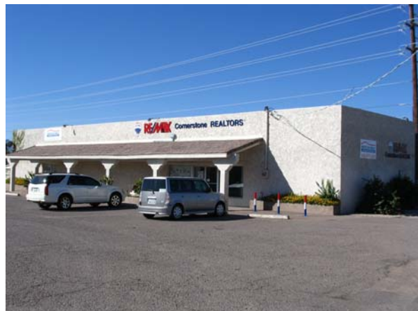
View looking southwest.
