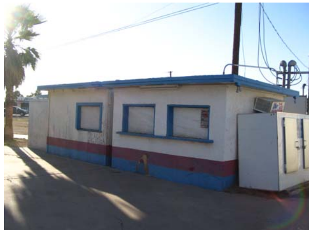
View of auxiliary concession stand, looking northwest.
