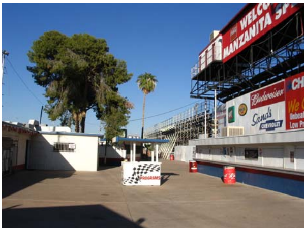
View of Entrance Plaza, looking east.
