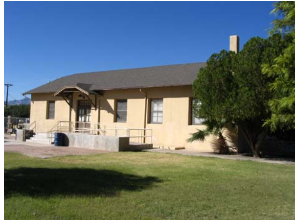
View looking southwest.
