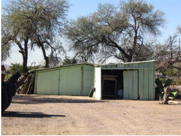
View of westernmost sheds (looking west).
