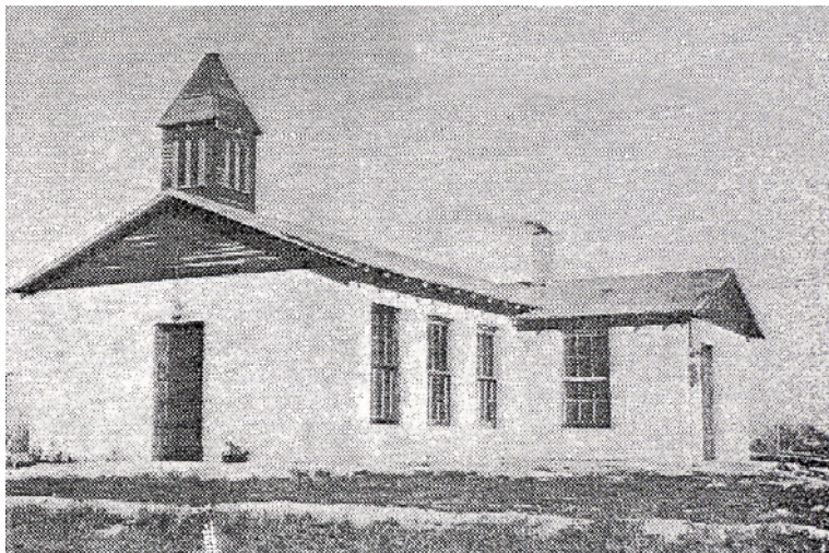
Figure 1.10 The original Laveen Baptist Church looking northwest from Dobbins Rd.
