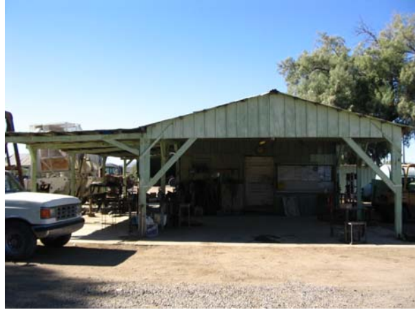
View of farm building (looking west).
