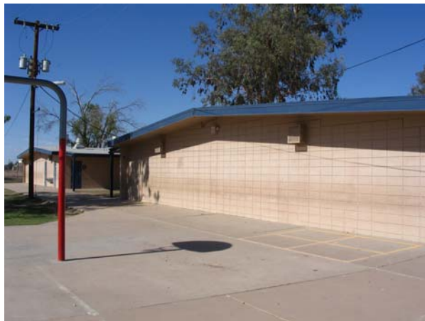
Rear school building with front building in background (looking northeast).
