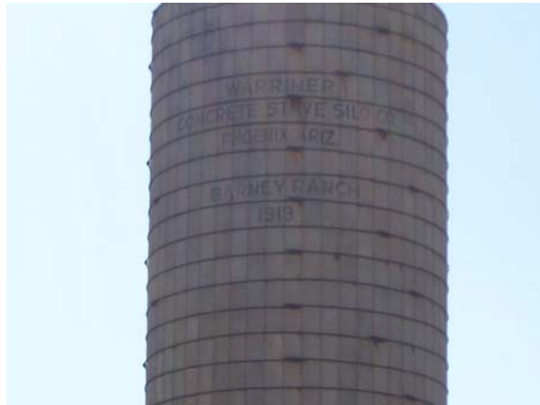
Farmstead silo with inscription: “Warriner, Concrete Stave Silo Co., Phoenix Ariz., Barney Ranch, 1919.”
