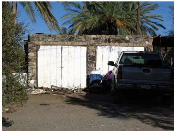
View of original garage looking east.
