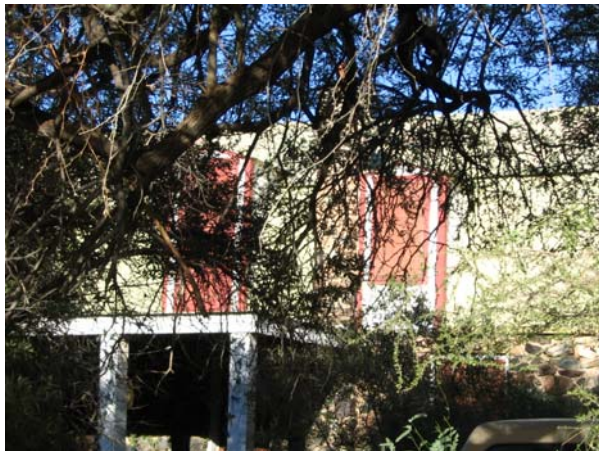
View of front façade, facing northeast.
