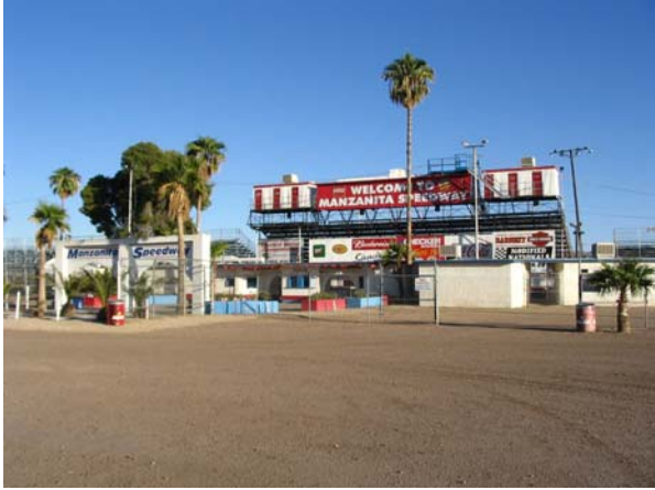
View of front facing southeast.
