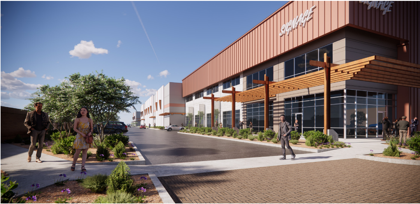
Building Character At South Elevation
