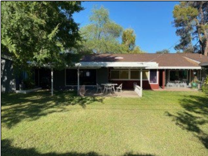
Photo 3. 8122 N 10th Ave, looking east
