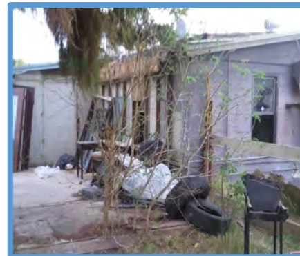
Code Compliance/ Abatement
