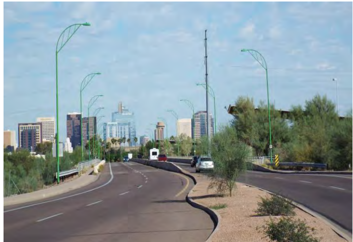
Central Avenue at the Audubon Center (view north).
