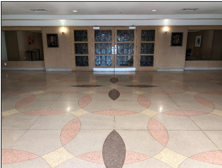
Photo 11. View of chapel doors and terrazzo floor in lobby, looking west from building entrance.
