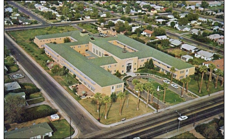
Photo 14. Early postcard showing aerial view of building (courtesy Reid Butler).
