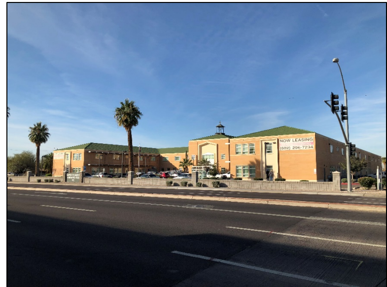
Photo 4. View of subject property, looking southwest across 16 th Street.
